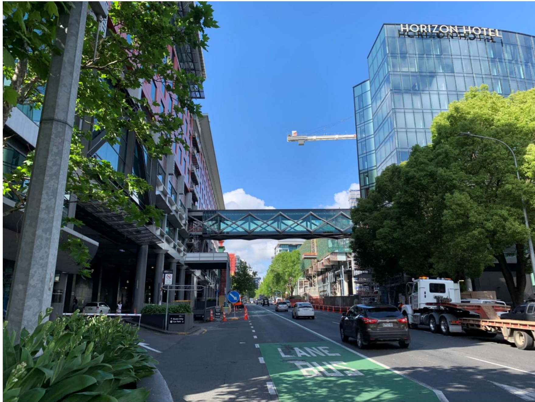
View from Hobson St – new linkway bridge
