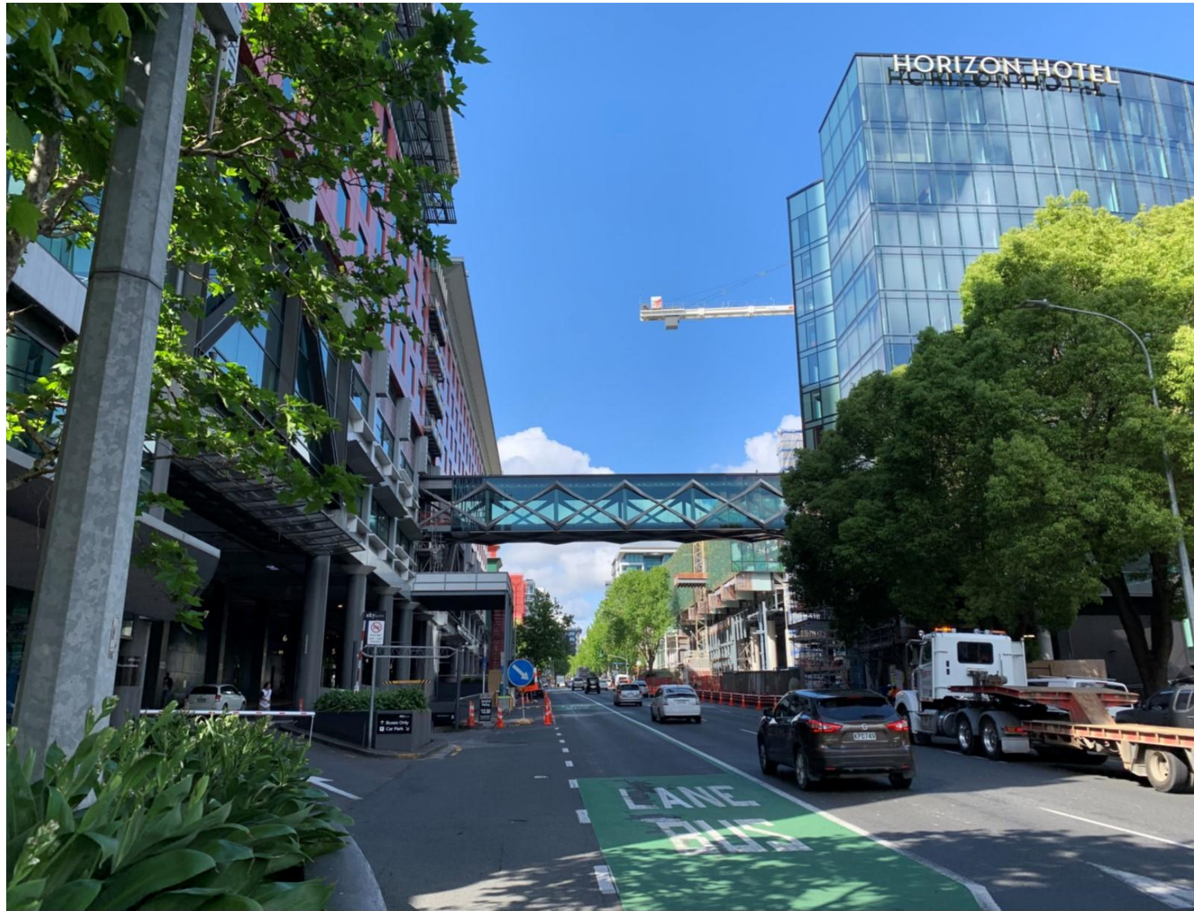
View from Hobson St – new linkway bridge
