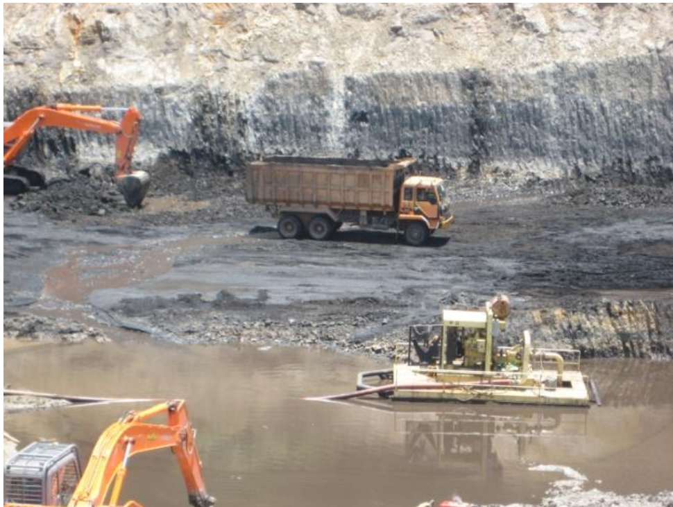
Pumping out of the Trinity pit at ADK
