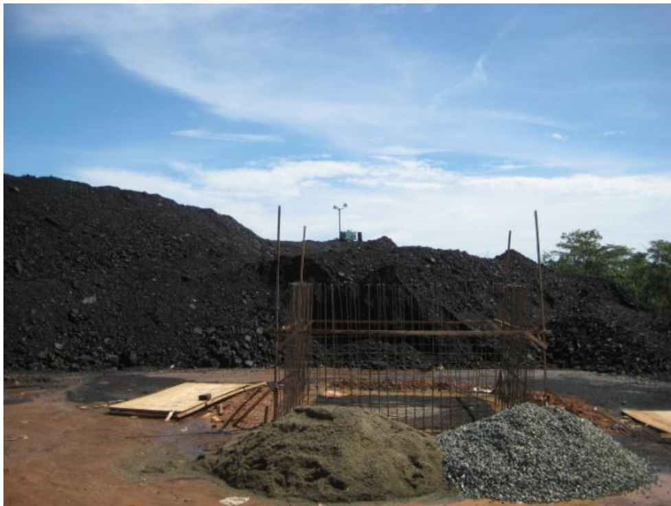
ADK stockpile in mid-October (approximately 40,000 tonnes) with crusher/weighbridge installation underway
