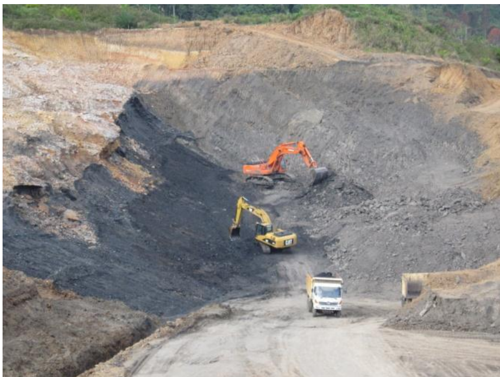
Exposing the coal seam and coal getting
