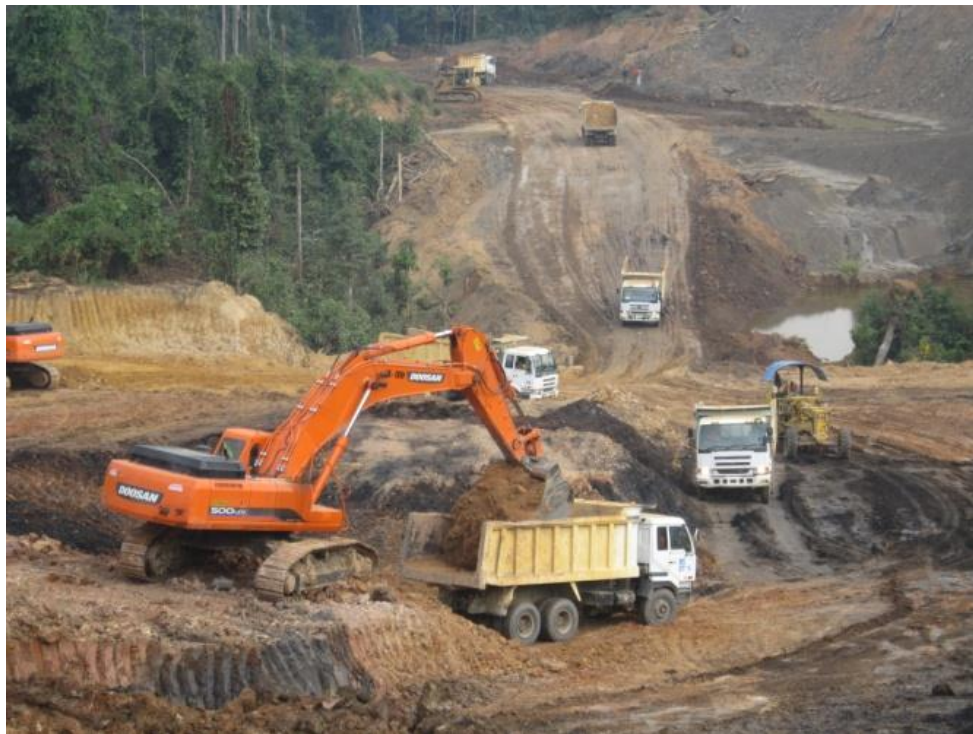
B2 overburden removal to expose coal seam(s).
