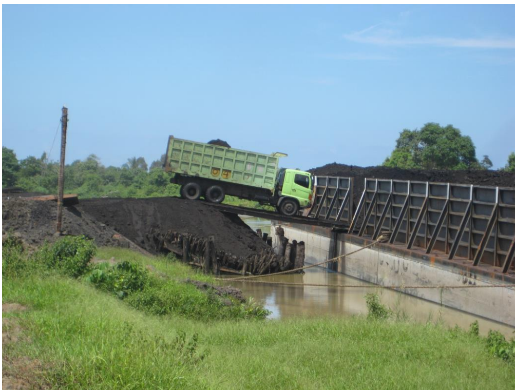
SKJM Port: Loading loading onto 5,000 tonne barge
