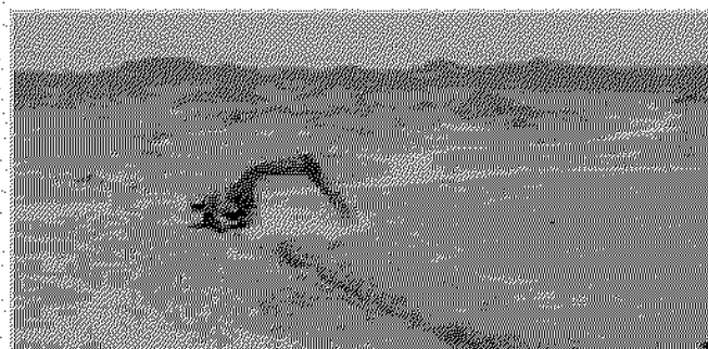
TRENCHING OF GEOCHEMICAL ANOMALIES AT HAIMUR
