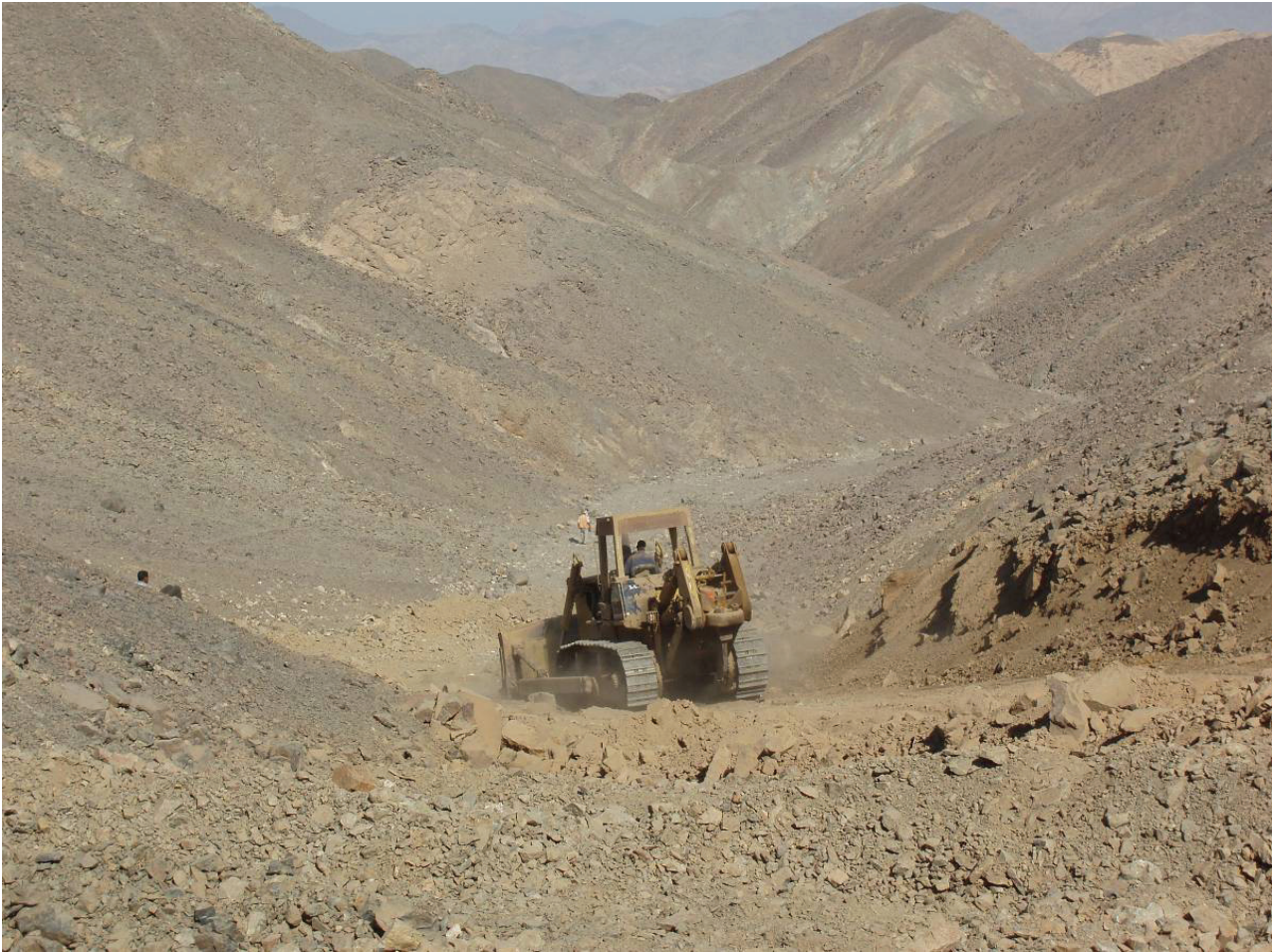
Figure 1: Construction of the Abu Dabbab mine access road
