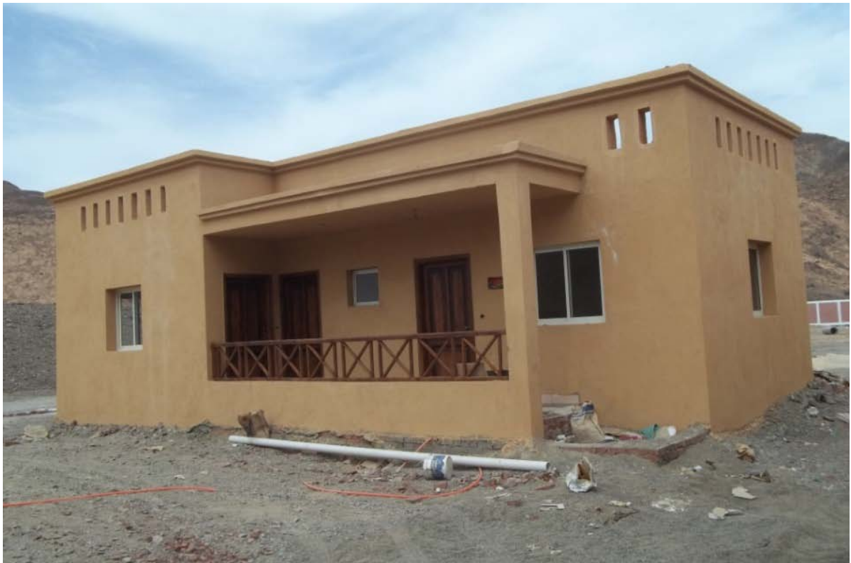
Figure 2: Customs house nearing completion
