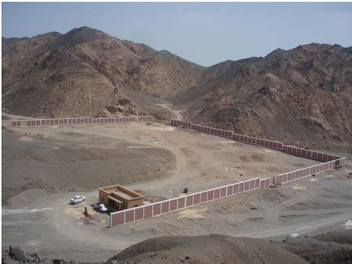
Figure 1: Free Zone compound, earlier shot showing brick walls and customs house; the walls on three sides are now completed.
