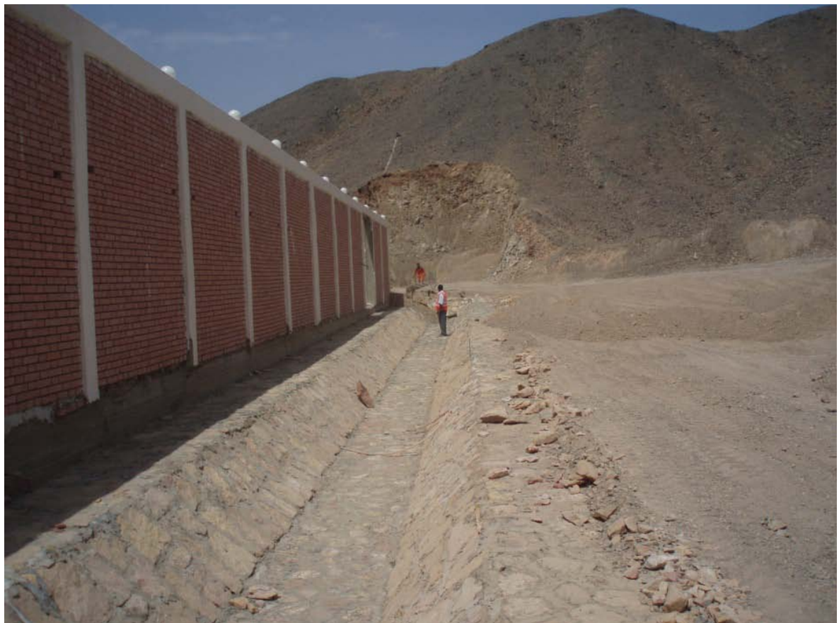
Figure 3: Drainage works around the FZ walls.
