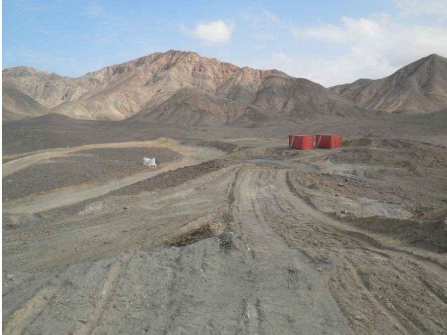
Figure 4: Pre-production earthworks at the ore processing site
