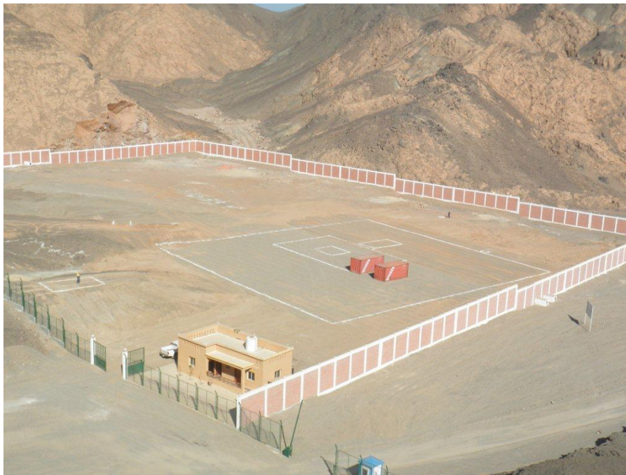
Figure 5: Floor mark-outs at the Free Zone finishing area following earthworks
