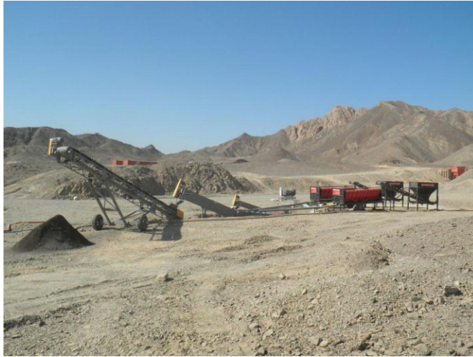
Alluvial Separator set up
