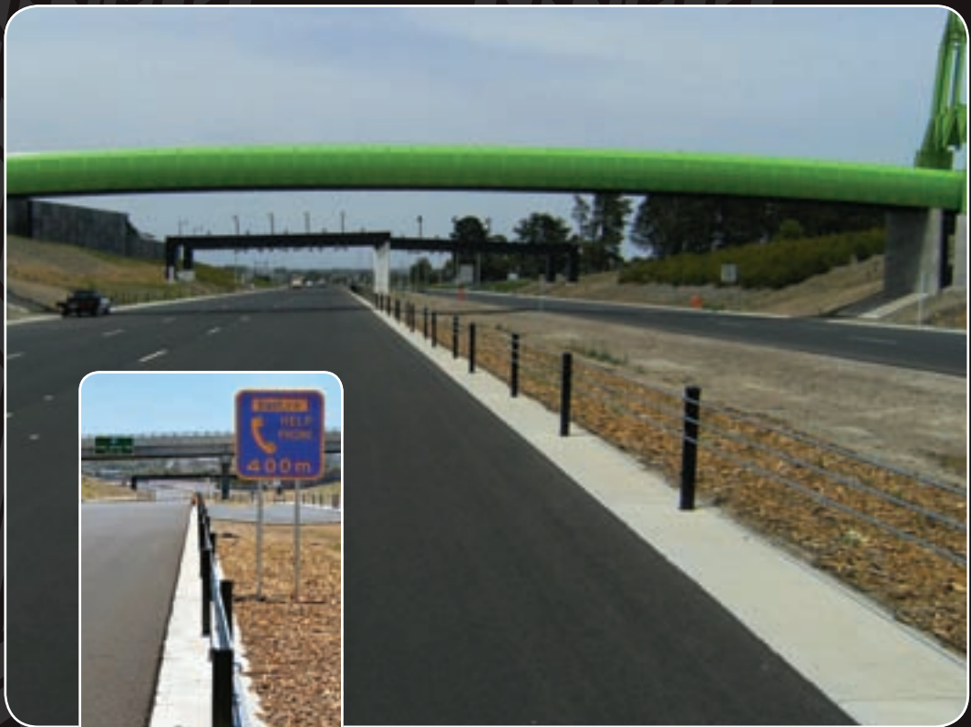
'Gibraltar' Wire Rope installation on Eastlink
