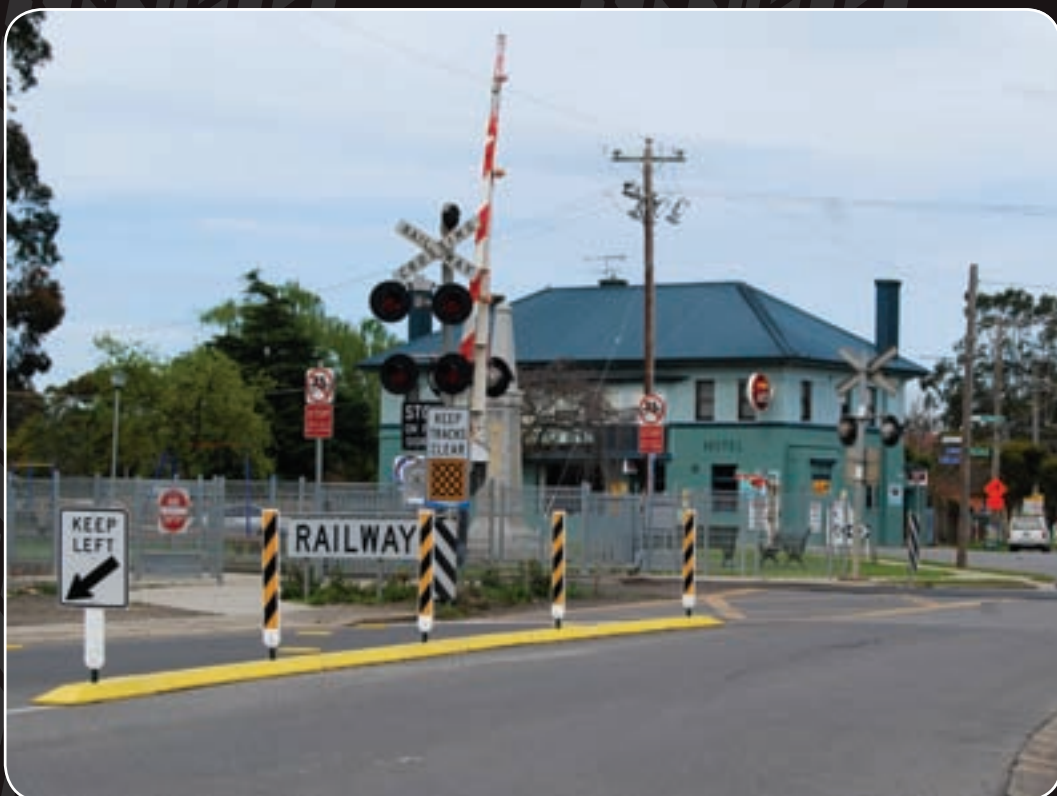
Separation Kerb with SnapLoc Guide Post and flexible sign at railway crossing
