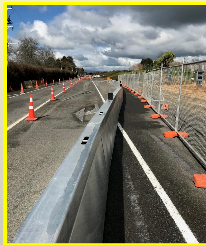
First HV2 Barrier installation in New Zealand
