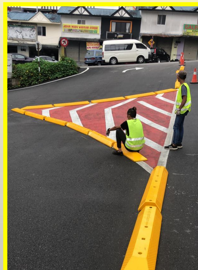
Separation Kerb in Malaysia
