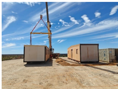
Plate 1: Installation of the Apollo Hill Development Camp
