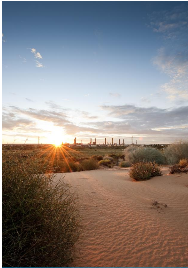
Moomba Plant, Cooper Basin
