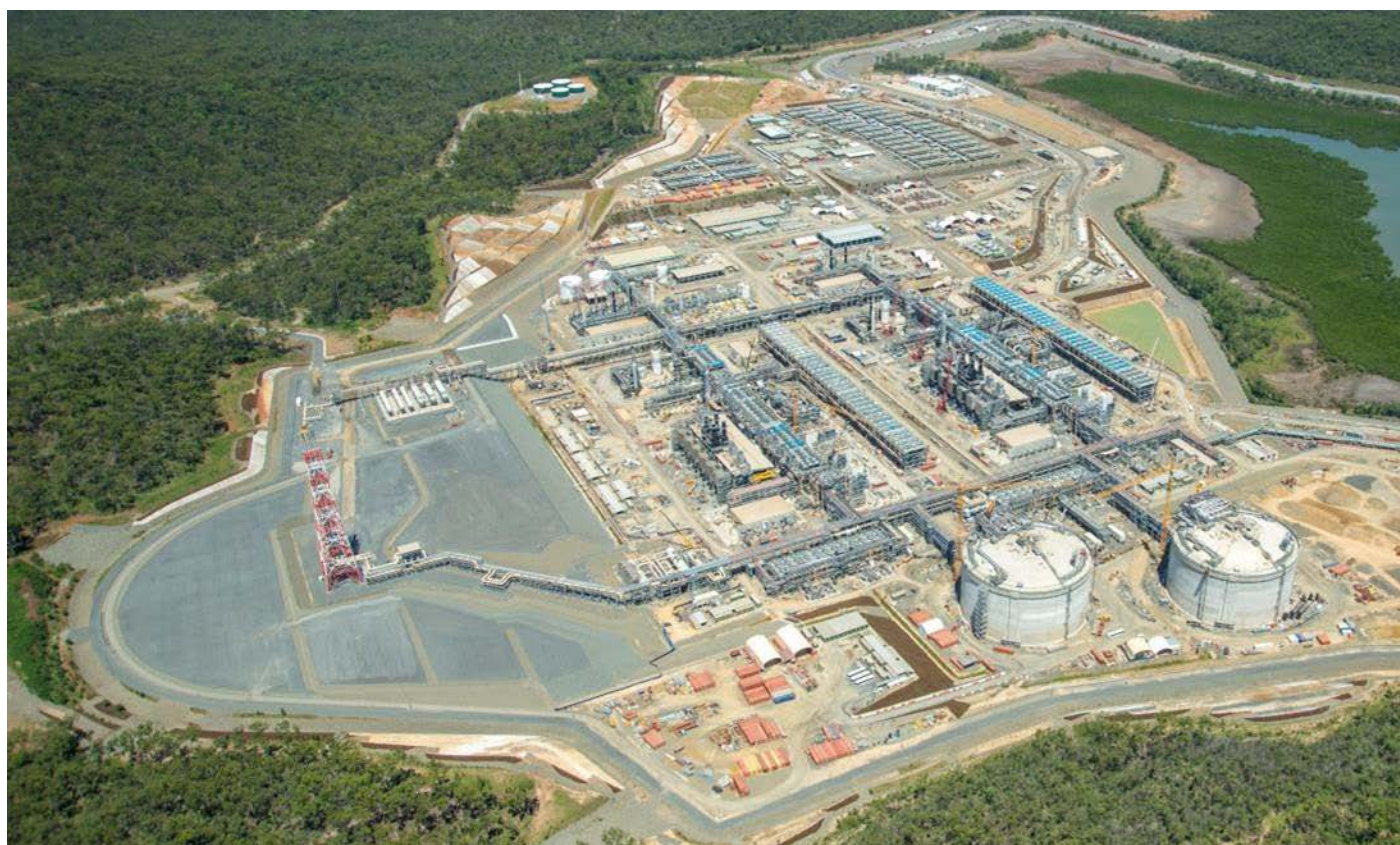
GLNG plant, Curtis Island, February 2015
