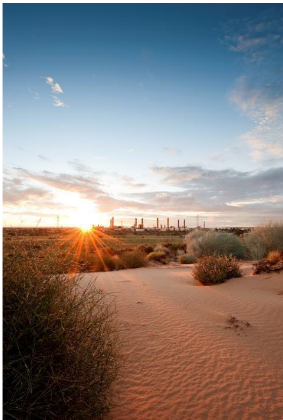
Moomba Plant, Cooper Basin
