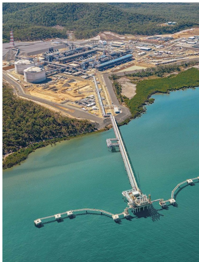
GLNG plant, Curtis Island, July 2015
