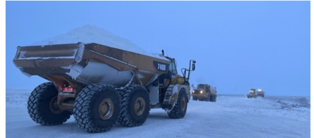
Ice road construction
