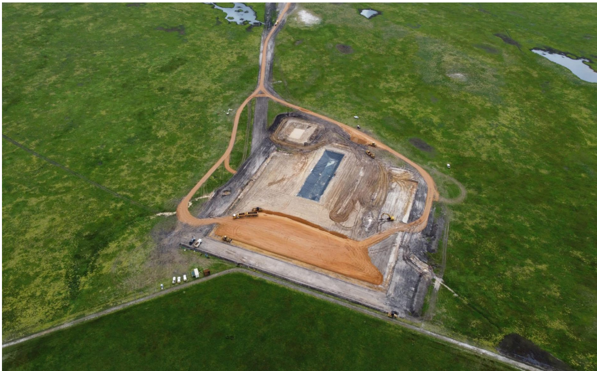
Walyering-5 well pad under construction
