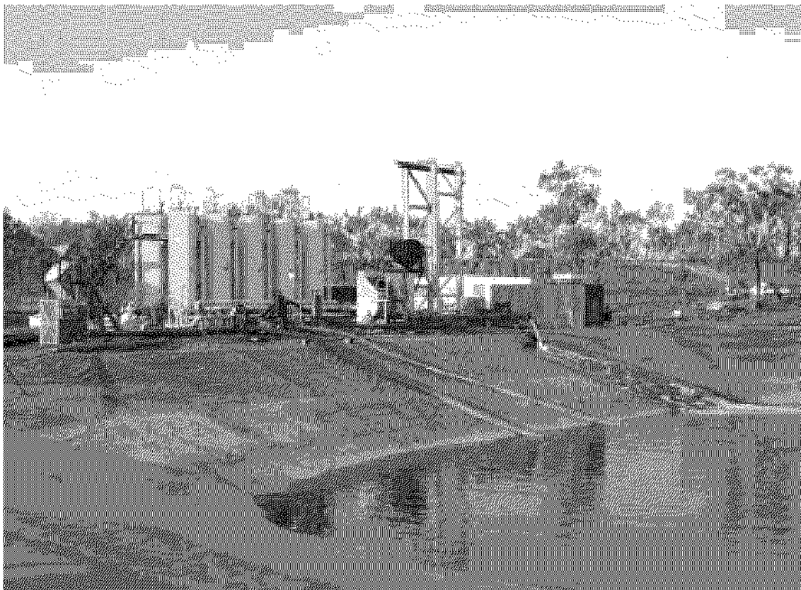
Quest 29 – Processing Plant
