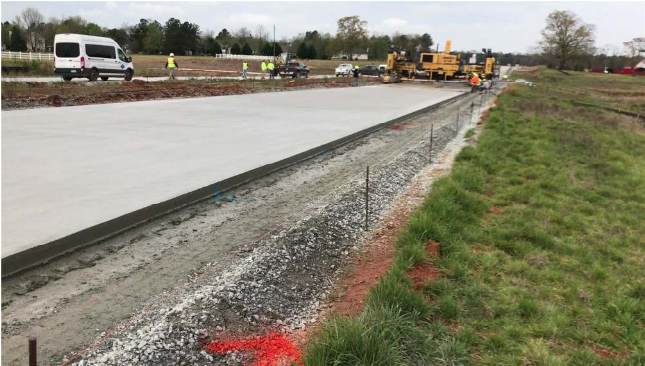
Figure 2. Completed section of highway with added EdenCrete®
