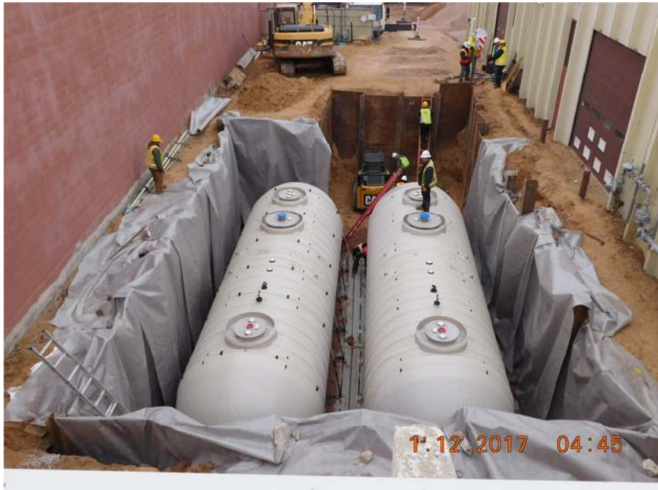
Figure 1. Two 20,000 gallons capacity EdenCrete™ underground storage tanks being installed (January 2017).
