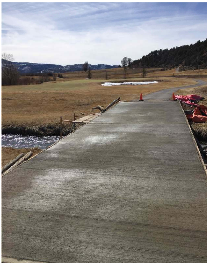
Figure 5. Gypsum Golf Course Bridge Project
