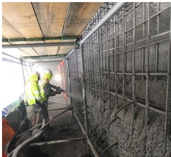
Figure 4. The EdenCrete® enriched Shotcrete being applied
