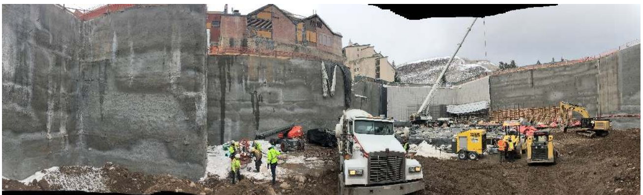
Figure 2. First section of final structural liner (centre - light grey area) being installed
