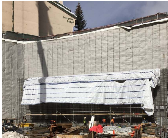
Figure 3. Site of installation of first 70 cubic yards of Shotcrete with EdenCrete®
