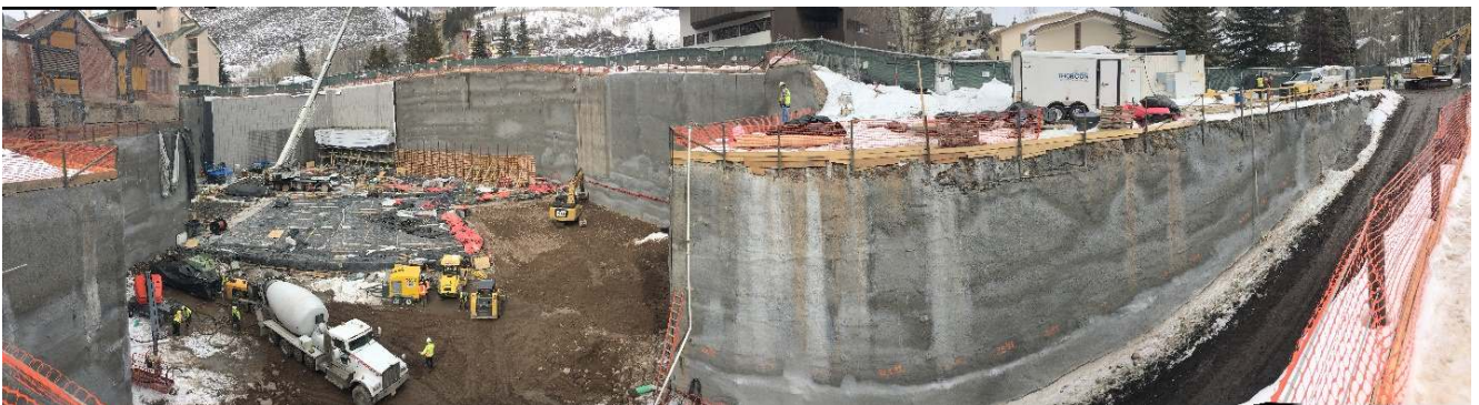
Figure 1. First section of final structural liner (top left- light grey area) being installed
