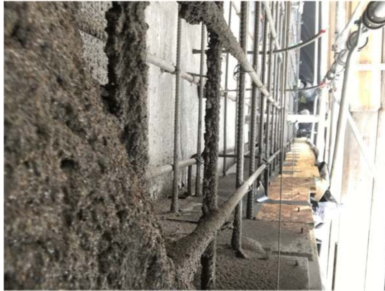
Figure 5. Close - up photo of EdenCrete® Shotcrete
