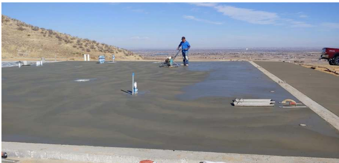
Figure 2. Finishing the concrete surface at the Loveland project
