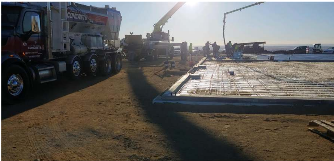
Figure 1. Volumetric truck mixing at the Loveland project site
