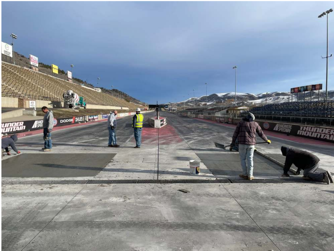
Figure 1. EdenCrete® concrete being placed in Burn Out Boxes
