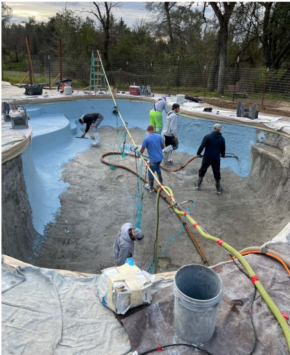
Figure 1. A typical US exposed aggregate, swimming pool finishing mix being applied in a trial in California.
