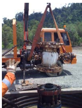
Figure 3 Removal of A-2 well head spool, to prepare for A-2 workover
