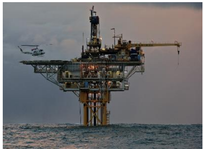
Cliff Head Alpha offshore platform
