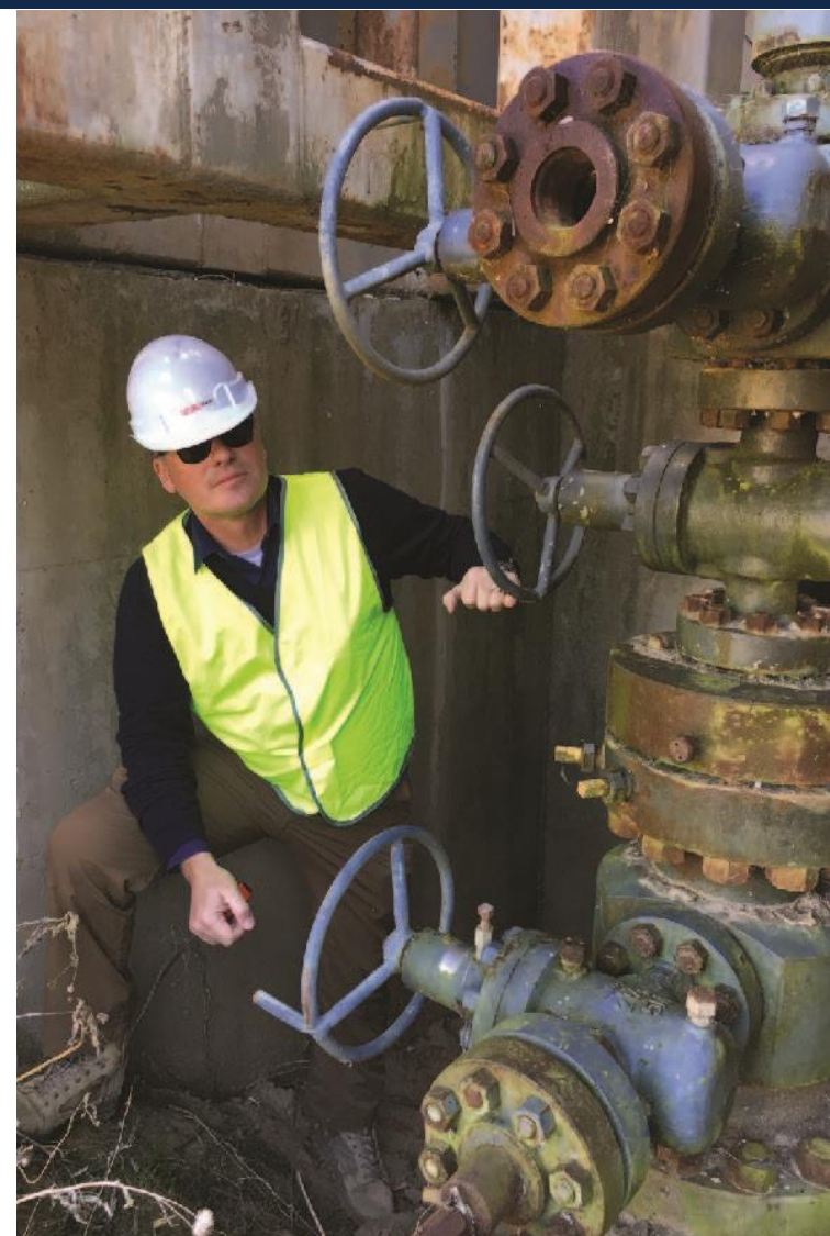
Primero-1 Wellhead in PL 231
