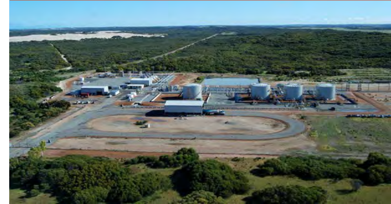
Arrowsmith Stabilisation Plant (ASP)
