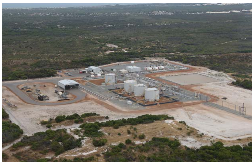
Arrowsmith Stabilisation Plant
