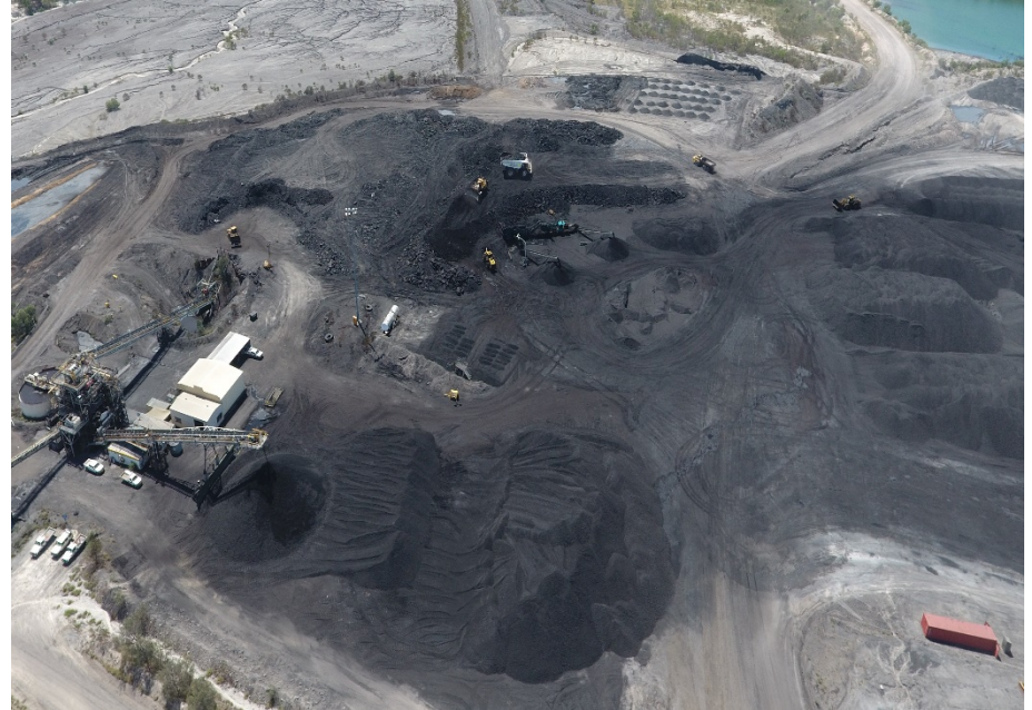
Blair Athol – CHPP and Stockpile.
