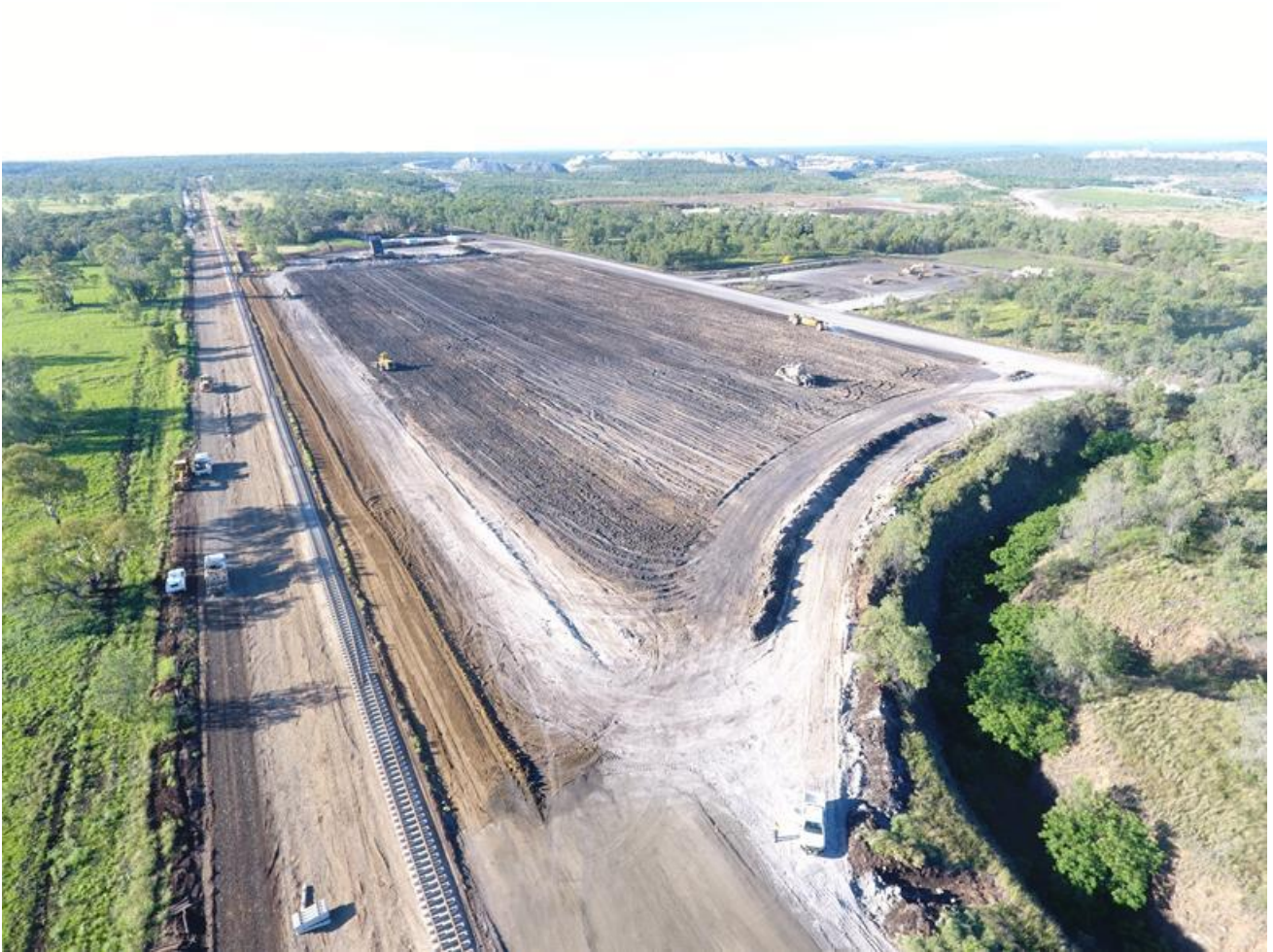
Figure 4 – BA Train Loadout and Rail Line Looking South
