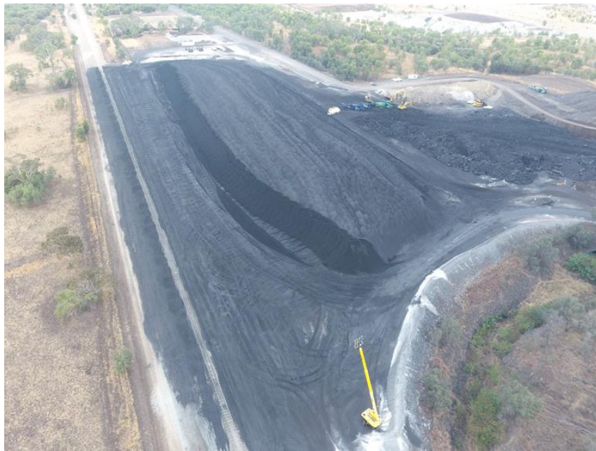
BA TLO Product Stockpiles with By-Pass Crusher System
