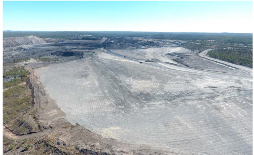
Image – Capped Tailings Dam
