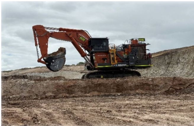
New EX3600-7 – First Bucket of Dirt
