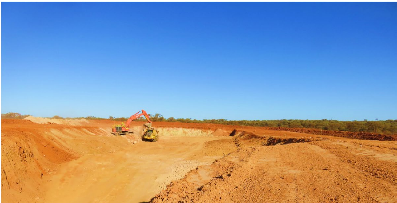
Figure 6: Monty boxcut development
