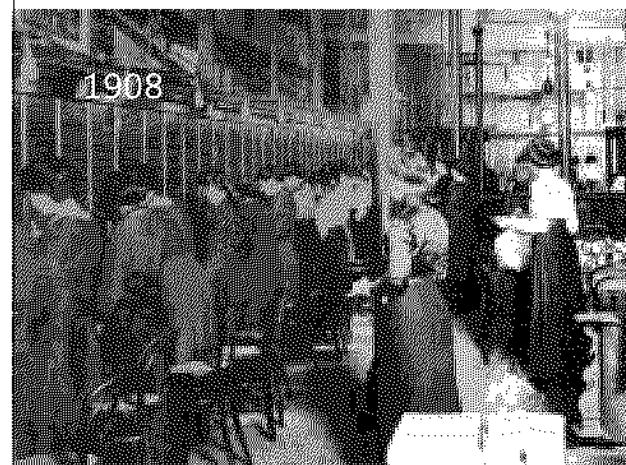
Telephone switchroom in PMG Exchange.
