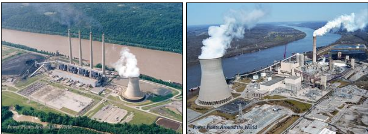
Figure 2: Typical Modern Scrubbed Coal Fired Power Plants on the Ohio River (Left: 2.4GW JM Stuart Plant, Right: 1.4GW Zimmer Plant)
