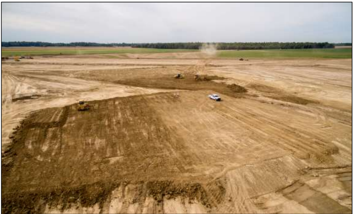
Site Pad Prepared for the Coal Handling and Preparation Plant ("CHPP") at Poplar Grove
