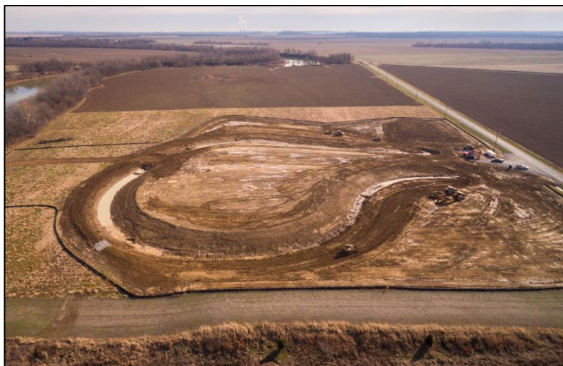
Accelerated site excavation at the Paringa barge load-out facility
