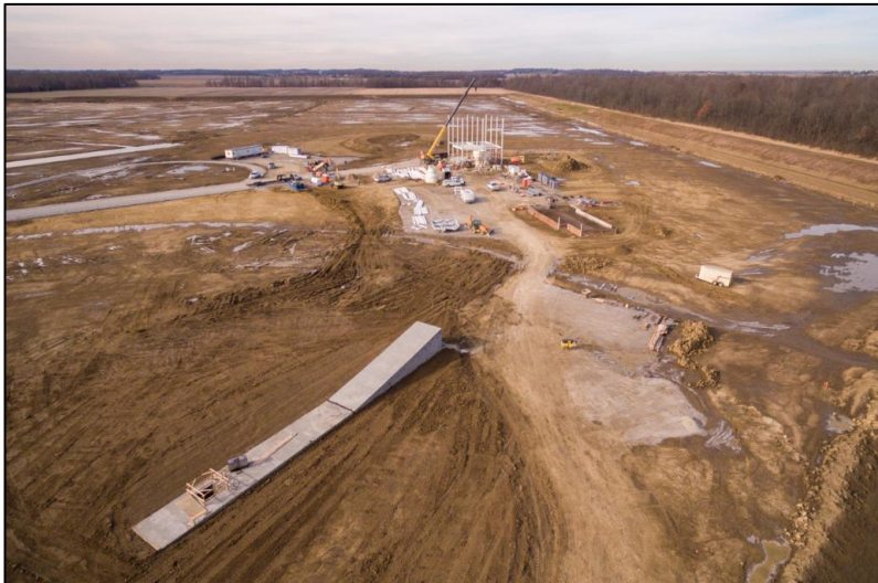
Completion of raw coal reclaim tunnel
