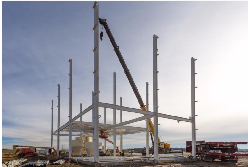
Erection of steel at the preparation plant
