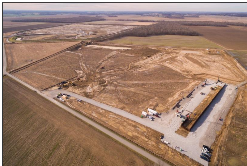
Construction of the keyhole slope decline to access underground coal
