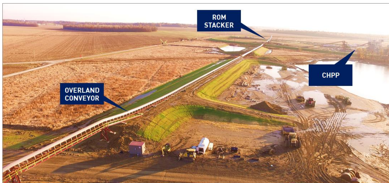
Figure 3: Overland conveyor from the mine to the CHPP nearing completion
