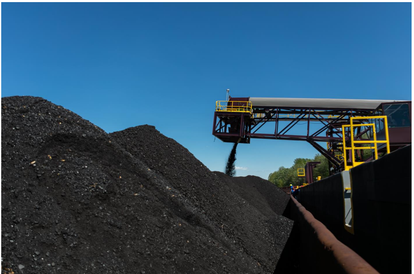
Figure 1: Barge loading operations at Paringa's Ainsworth Dock on the Green River
