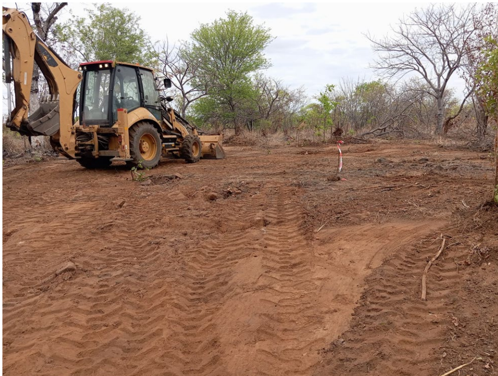
Figure1 – Initial site preparation undertaken at Aucu, including light clearing and grading to establish access for early field activities.
