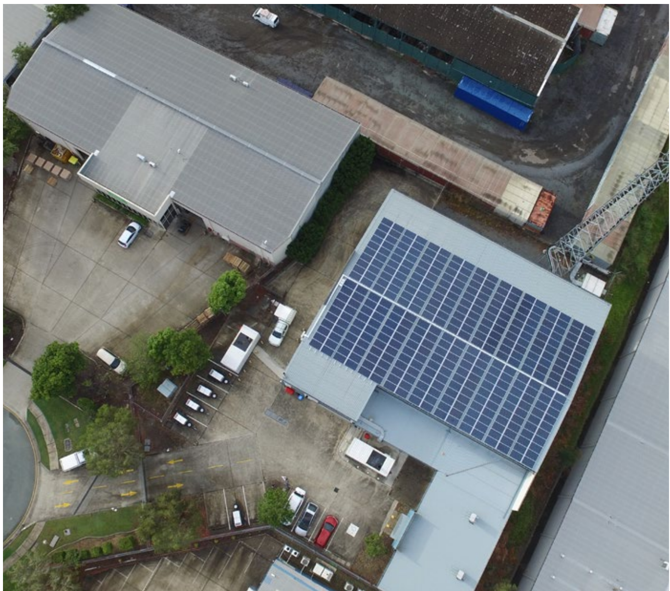
Solar power on-site at Labrador, Queensland.
