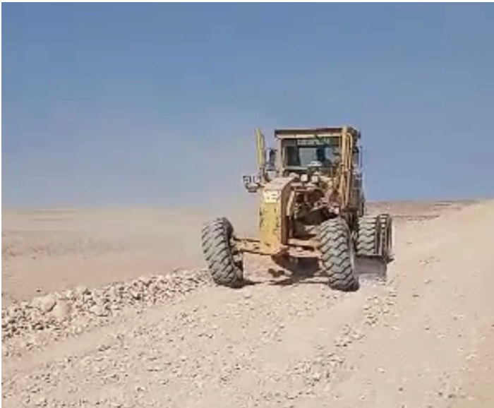
Figure 3: Work on access track improvements in-progress.
