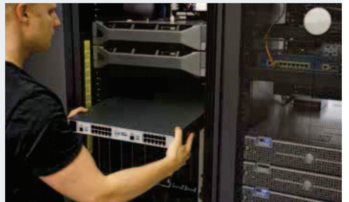
> TZ IXP Praetorian™ Junction installation.
