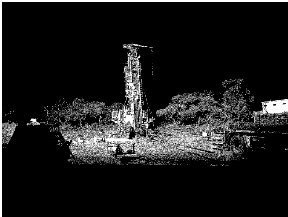
Drill Rig at Menninnie Dam (MD54 July 2006)
