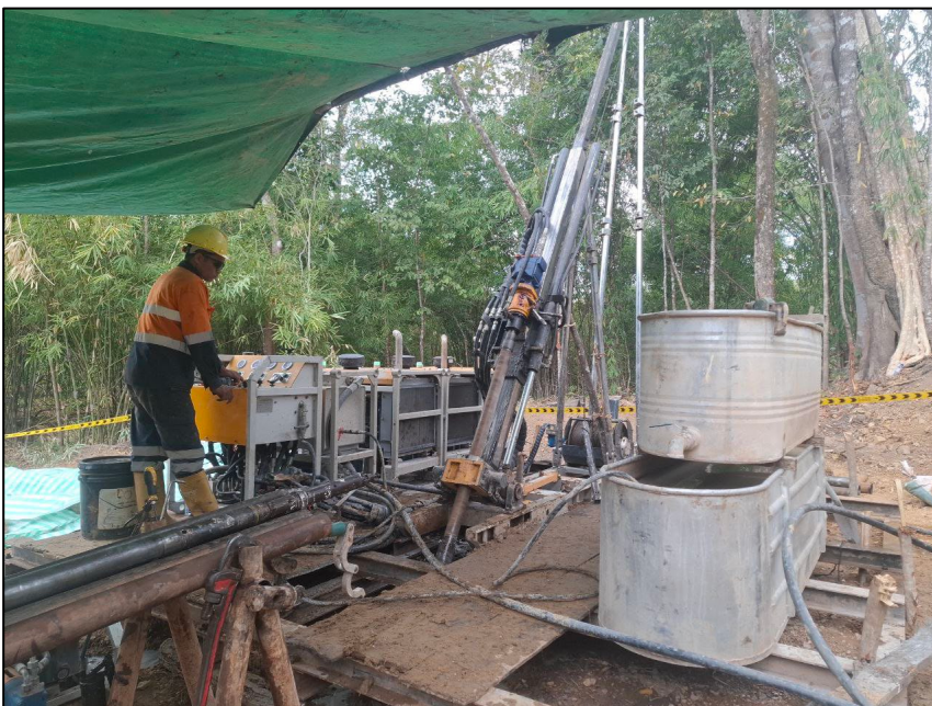
Figure 1: Second drilling rig underway at Ngot
