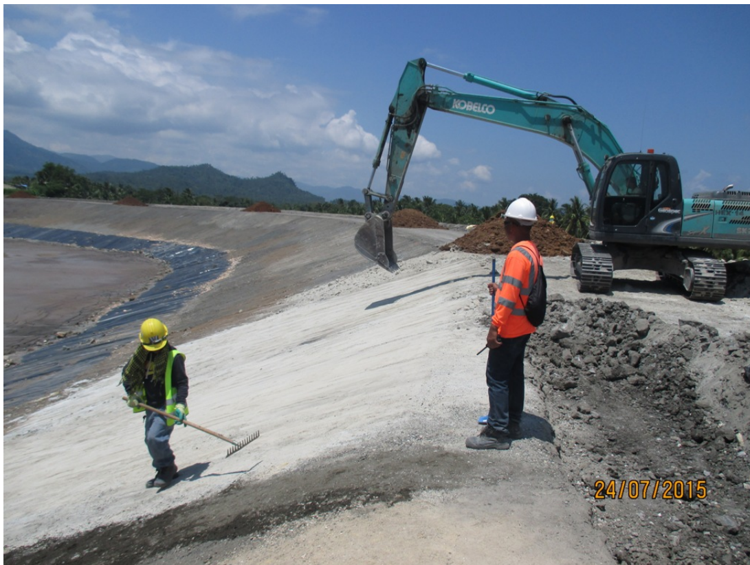
Figure 4: HDPE Tailings Storage Facility construction
