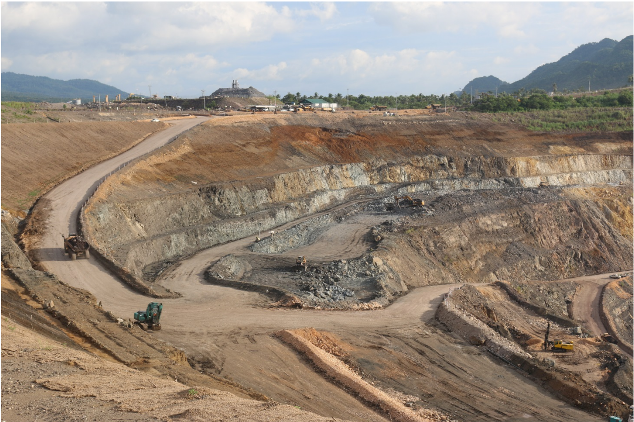
Figure 1 – Siana open pit Western wall cut-back with the ROM pad, site offices and power station in the background
