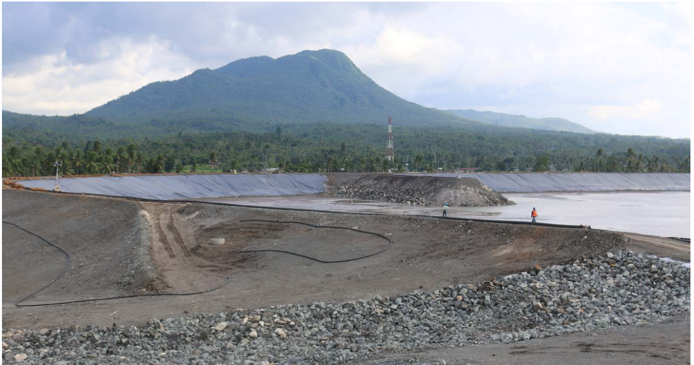
Figure 3 – Tailings Storage Facility 5 (HDPE TSF5) showing the HDPE lining
